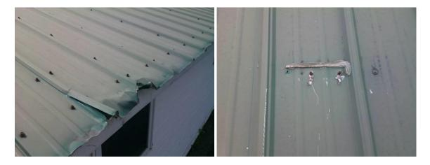
Corrugated metal roof panel fasteners (nails and/or screws) can work loose over time and lose their seal. Care should be taken to tighten/replace fasteners where loose. I noted
