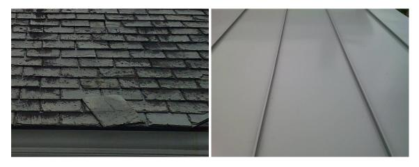
The standing seam metal roof covering over the rear (east) portions of the structure appeared moderately weathered, in a manner consistent its age. One might reasonably many (five plus) years remaining serviceable life.
