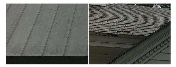
I noted the potential for wintertime ice and snow build-up at roof valleys and pitch changes. Manual snow removal at these areas can help control ice dams. Also, I recommend installing a cap at the south chimney to help prevent water, pest and debris entry into the flue, and to reduce chimney deterioration over time.
