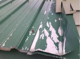
I noted bent metal panels at the west wall porch roof. This is likely caused by snow and ice falling from the roof above. The panel damage does not appear to be causing roof leaking, and as such should not be considered an immediate deficiency. Panel replacement is possible, but keep in mind that the situation will likely re-occur because of snow and ice in future years, and may therefore not be seen as worthwhile.
