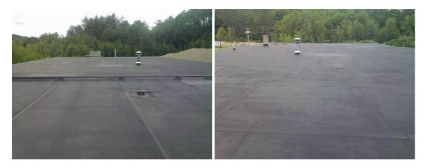
During my inspection, I found the rubber membrane roof covering to be moderately weathered, in a manner consistent with its age. One might reasonably expect at least several (three to five) years remaining serviceable life, with need for replacement increasingly likely thereafter.
