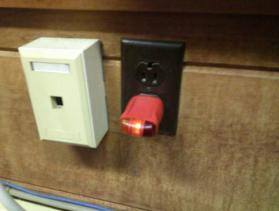
As a general rule, I recommend the eventual upgrading of all ungrounded circuits. This involves installing new wiring to fixtures at various locations throughout the building, and can be an expensive improvement.
