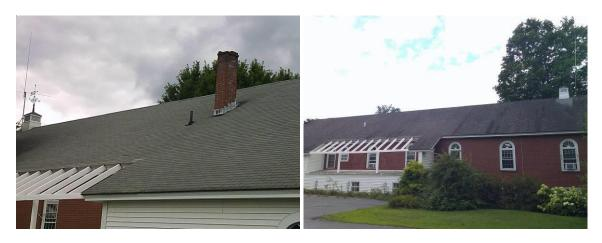
During my inspection, I found the asphalt shingle roof covering to be moderately weathered, in a manner consistent with its age. One might reasonably expect several (three to five) years remaining serviceable life, with need for replacement increasingly likely thereafter. The rubber membrane roof coverings appeared in good condition, with many more (five plus) years remaining serviceable life to be expected.
