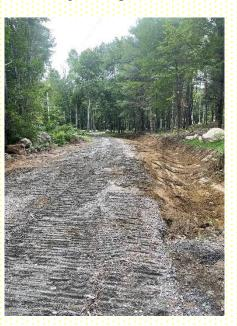
The Highway Department began a new project on South Mountain Road on September 1<sup>st</sup>. As you can see in the picture on the left the road has narrow ditches and erosion. The middle and right pictures show the next stage in the process to create ditches for proper drainage.
