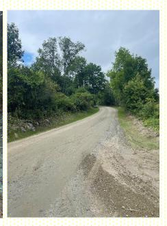
After the ditches are complete and culverts installed our Highway Department seeds all disturbed areas to eliminate erosion. The left and middle picture is Gulf Road and the picture on the right is Piper Road.
