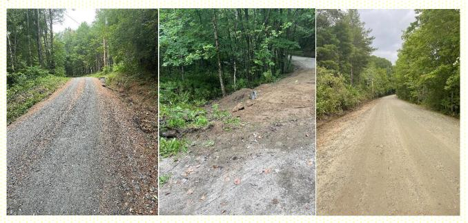
The picture on the left (South Mountain Road) shows a road with narrow ditches, which causes erosion and road washouts. As you can see on the right side of the road, water runoff has caused washouts in the road. When a road washes out it takes away the gravel.
