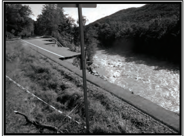
Collapse of Route 106 south of Downers from Tropical Storm Irene. Photo by Jim Mullen
